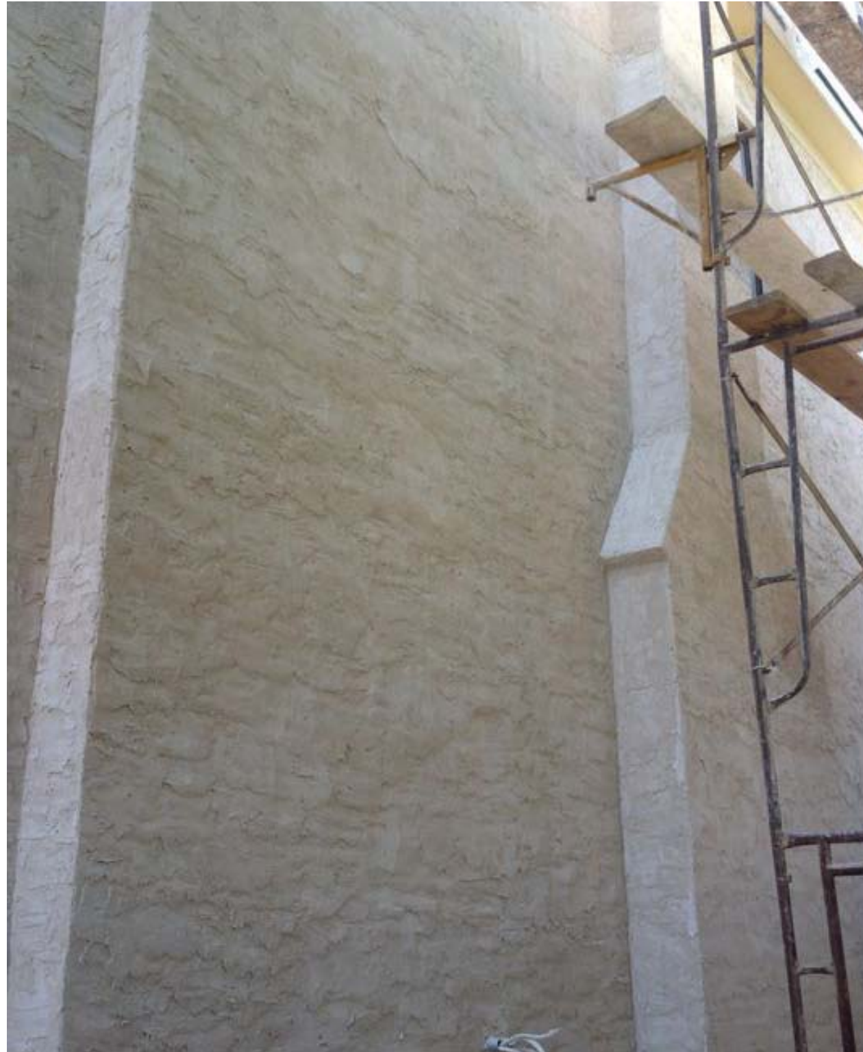
PARGED / FILLED MASONRY & TEXTURED INVESTIGATION
